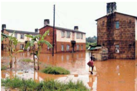
Plate 3.1: A flooded housing Estate constructed in a wetland
